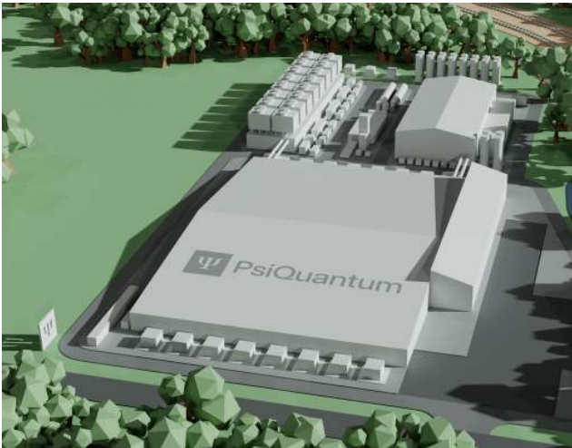
Figure 314: PsiQuantum map of their upcoming Brisbane facility with a cryoplant, a compute building to host their 100 logical qubit QPU, a research and office building. Right, two cryogenic casing for PsiQuantum's QPU. Construction began in June 2026 after over a year of delay. The Linde cryoplant will be installed in mid-2027 and the first cabinets afterwards. Source: [2794].
