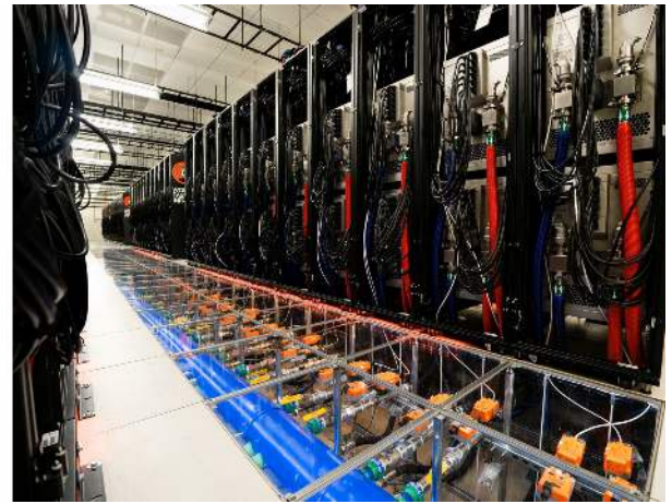
Figure 20: The Cerebras-based datacenter built in Oklahoma City in 2025 with 350 Cerebras chips and a peak performance of 40 exaflops of AI compute for a 10 MW power draw. Source: [54].
