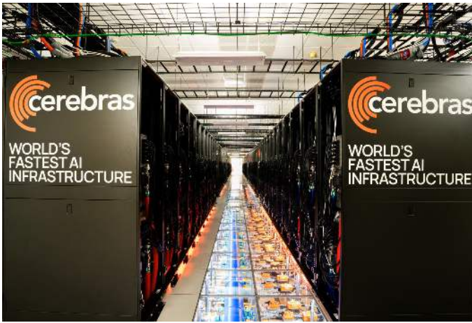
Figure 20: The Cerebras-based datacenter built in Oklahoma City in 2025 with 350 Cerebras chips and a peak performance of 40 exaflops of AI compute for a 10 MW power draw. Source: [54].
